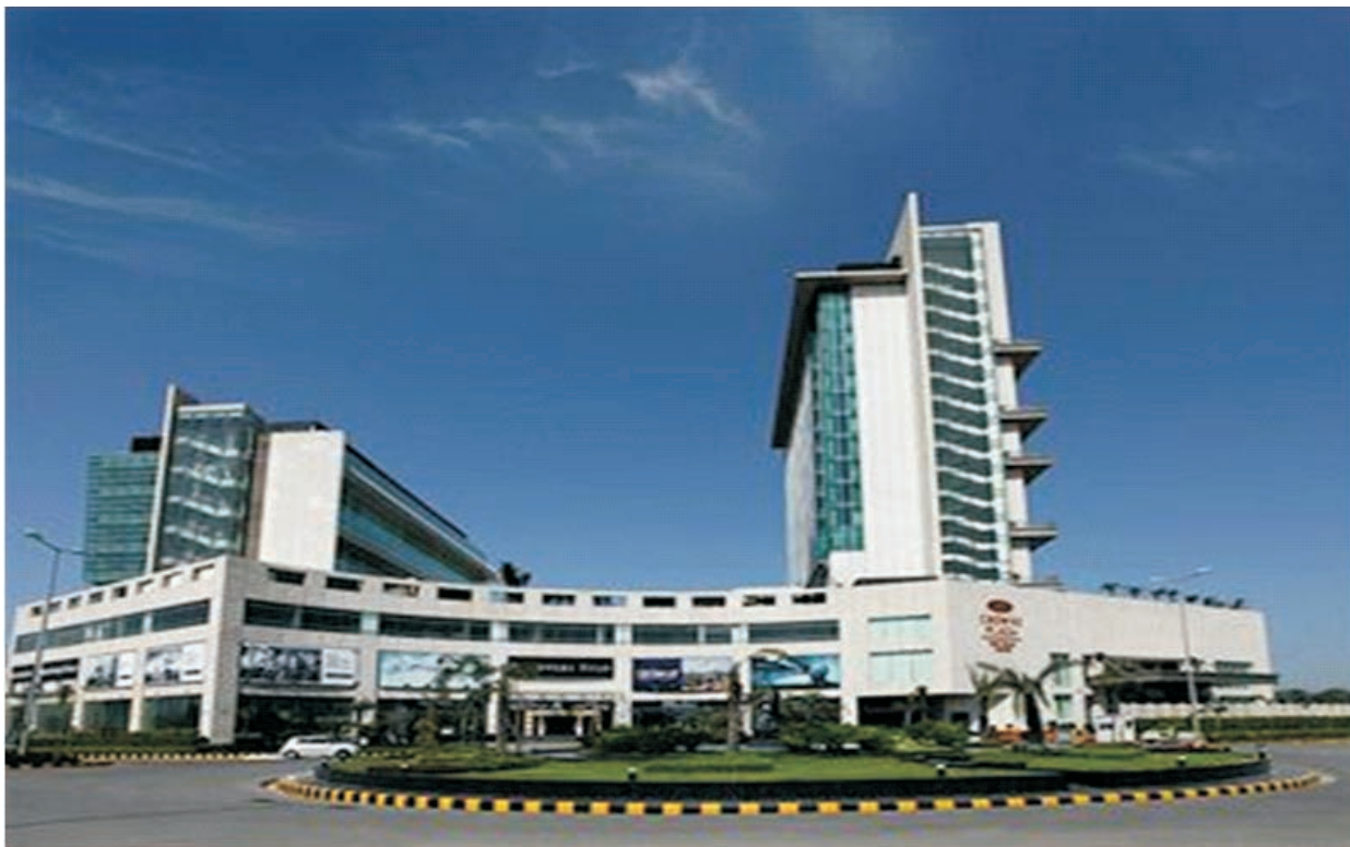
ROHINI—TWIN TOWER DISTRICT CENT (Rohini)
